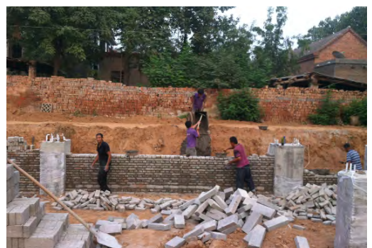
Church construction project in the Province of Hebei.
